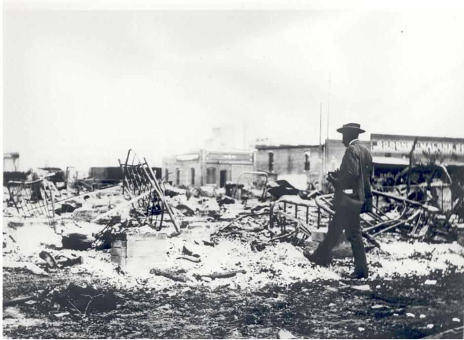
Destruction from the Tulsa Race Massacre (15583.B, Oklahoma Historical Society Photography Collection, OHS).
