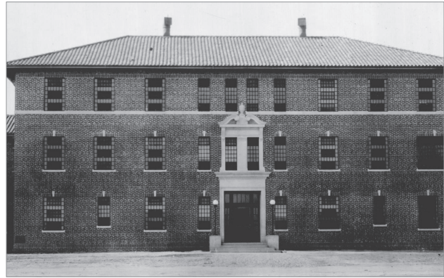
Exterior of the Taft State Hospital for the Negro Insane, 1936 (2012.201.B0266.0318, Oklahoma Publishing Company Photography Collection, OHS).
