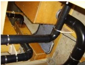
The motor compresses air and puts it into a closed system of ducts called **windlines**, which transfer the air to the organ chambers.
