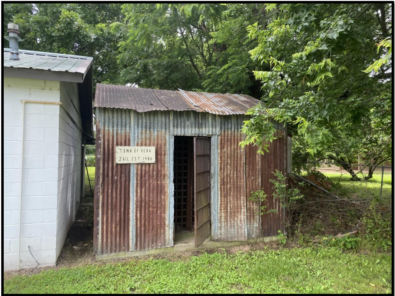
Figure 10: Vera Jail, Washington County. Build date ca. 1906. The Vera jail is the only known extant metal cell housed in a wood-frame iron-clad exterior. It was moved in 1991 roughly six blocks from its original location to protect it from further vandalism.
