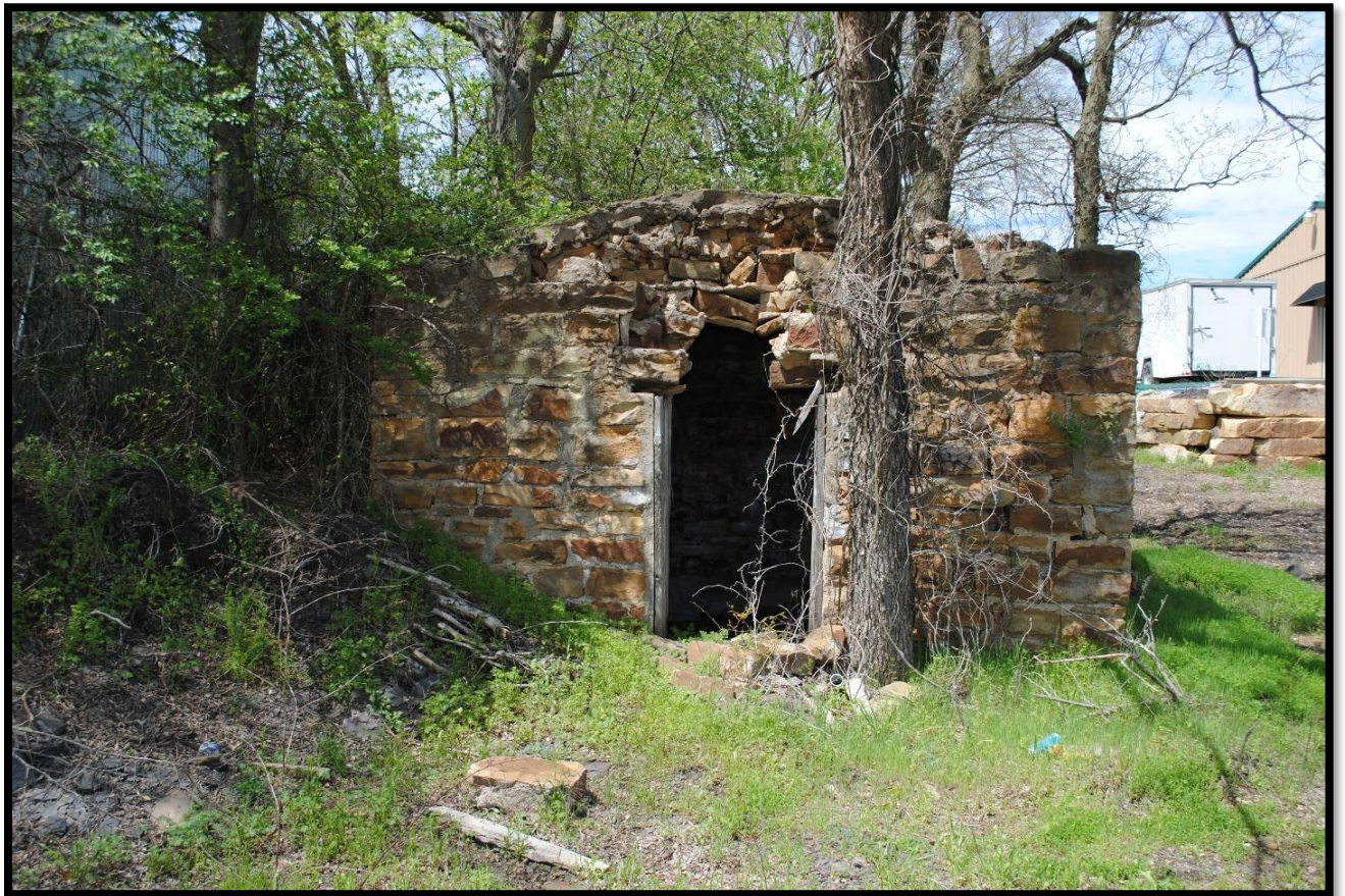
Figure 2: Keota Jail, Haskell County. The build date is unknown. One-room native stone. Barrel roof with ventilation openings at side elevations.
