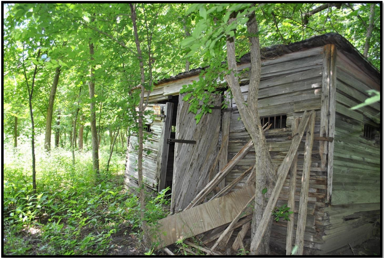
Figure 1: Skedee Jail, Pawnee County. Build date 1904. Two-room calaboose with separate entry doors for each cell. Stacked 2"x4" exterior with ventilation openings with iron bars at front and side elevations. Corrugated metal is used for the roof.
