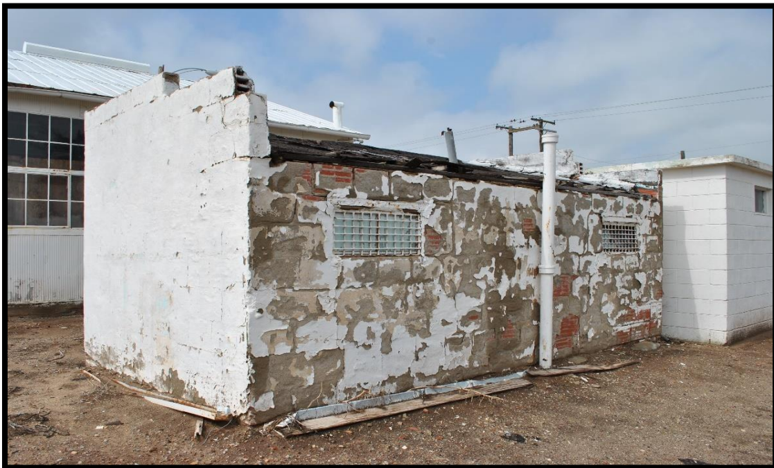
Figure 8: Laverne Jail, Harper County. Build date 1930. Two-room clay tile exterior, flat roof with a stepped parapet, and an additional front interior corridor area.
