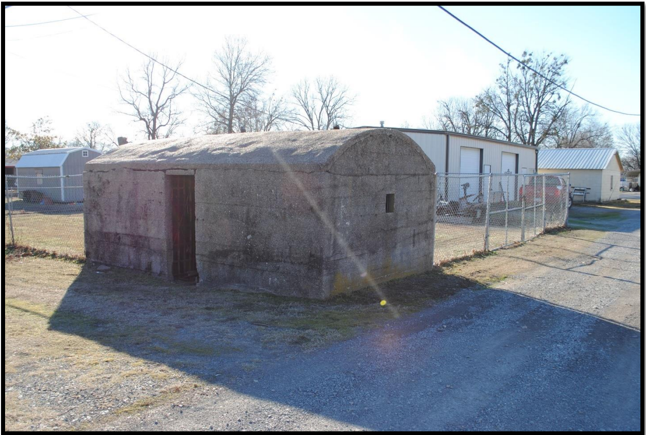
Figure 5: Chouteau, Mayes County. Build date ca. 1920. Two-room formed concrete. Barrel concrete roof. Single entry door with a small interior corridor separating the two cells. Small ventilation openings at the sides and rear for both cells.
