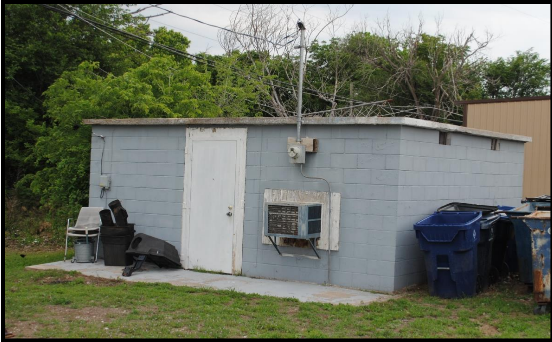
Figure 7: Longdale Jail, Blaine County. Build date unknown. Two-room concrete block exterior, flat concrete roof, and additional front interior corridor area.
