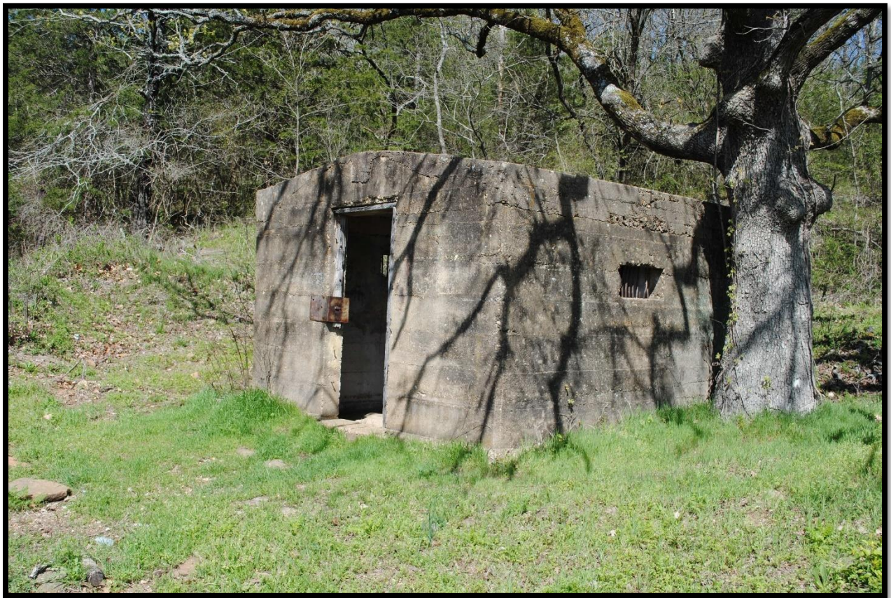
Figure 3: Marble City Jail, Sequoyah County. Build date ca. 1911. One-room formed concrete. Barrel roof with ventilation openings at side elevations.
