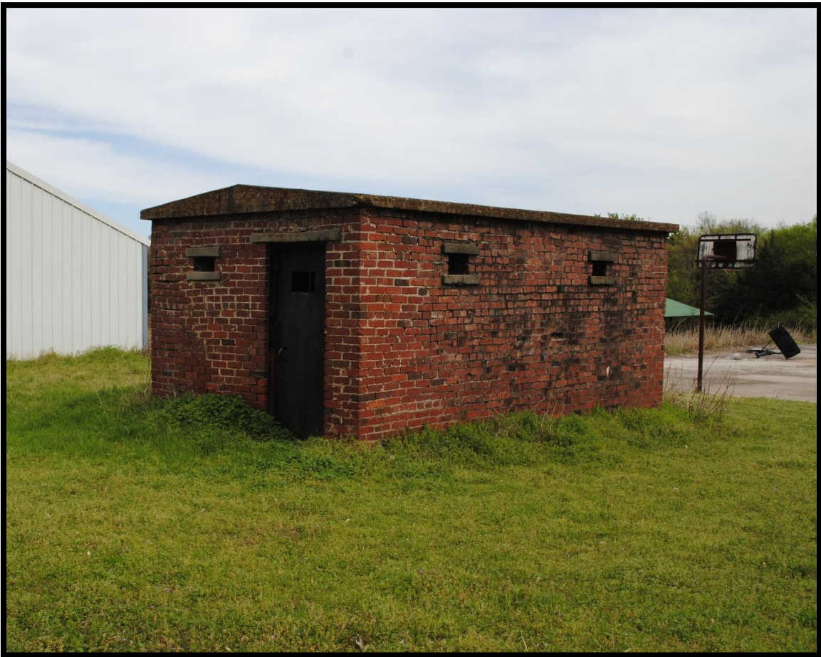
Figure 6: Canadian Jail, Pittsburg County. Build date pre-1907. Originally a two-room jail. One interior wall has since been removed. Listed on the NRHP in 1979 as part of the Canadian jail and livery stable.
