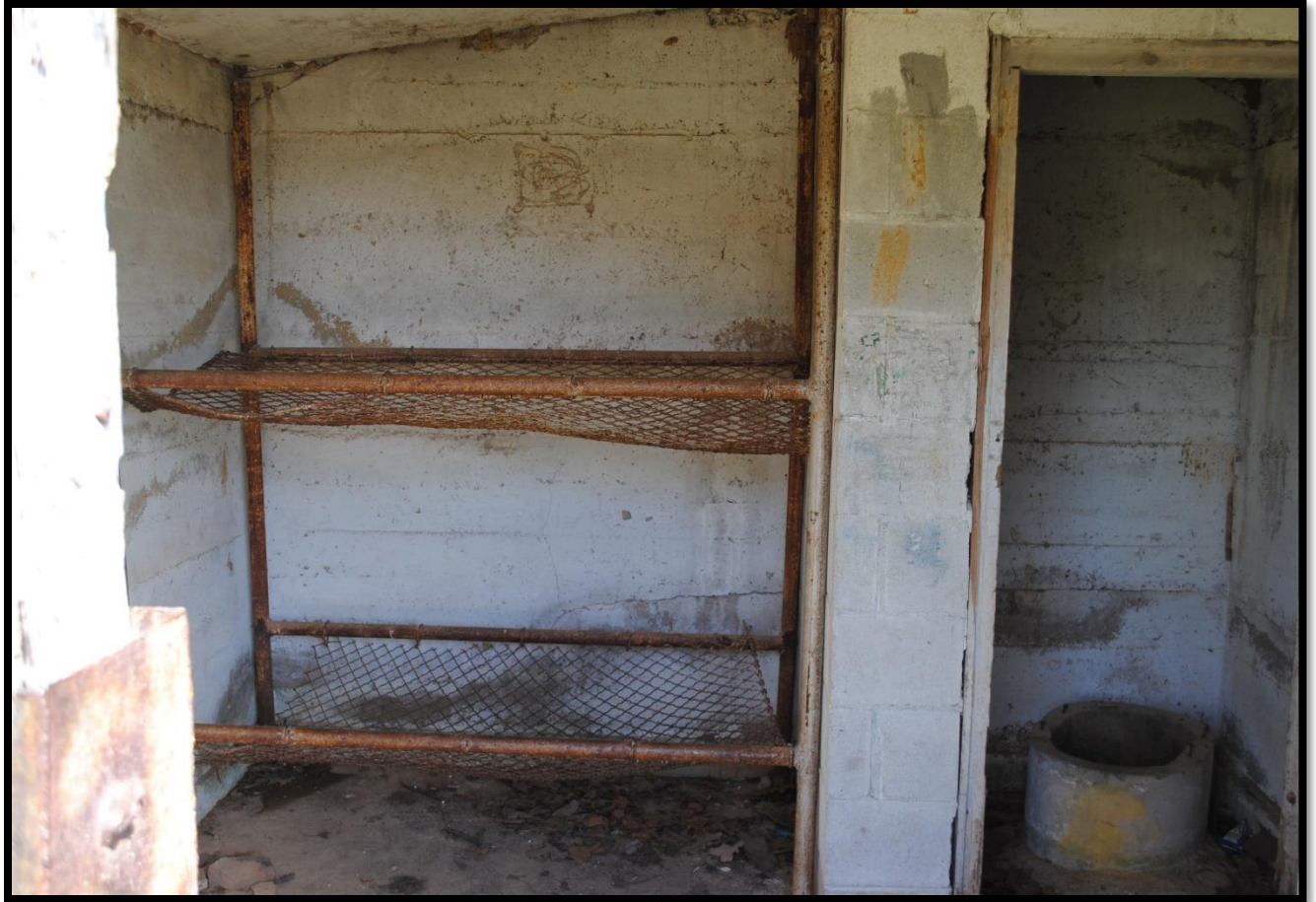
Figure 4: Interior view of Marble City Jail, Sequoyah County. Two bunks with a concrete latrine separated by a concrete wall.
