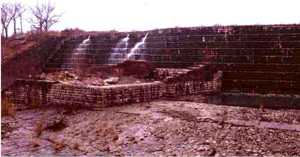
Image 6. Lake Okmulgee Dam and limestone spillway, constructed by the WPA. Reproduced from http://nr2_shpo.okstate.edu/images/98001591/98001591.jpg
