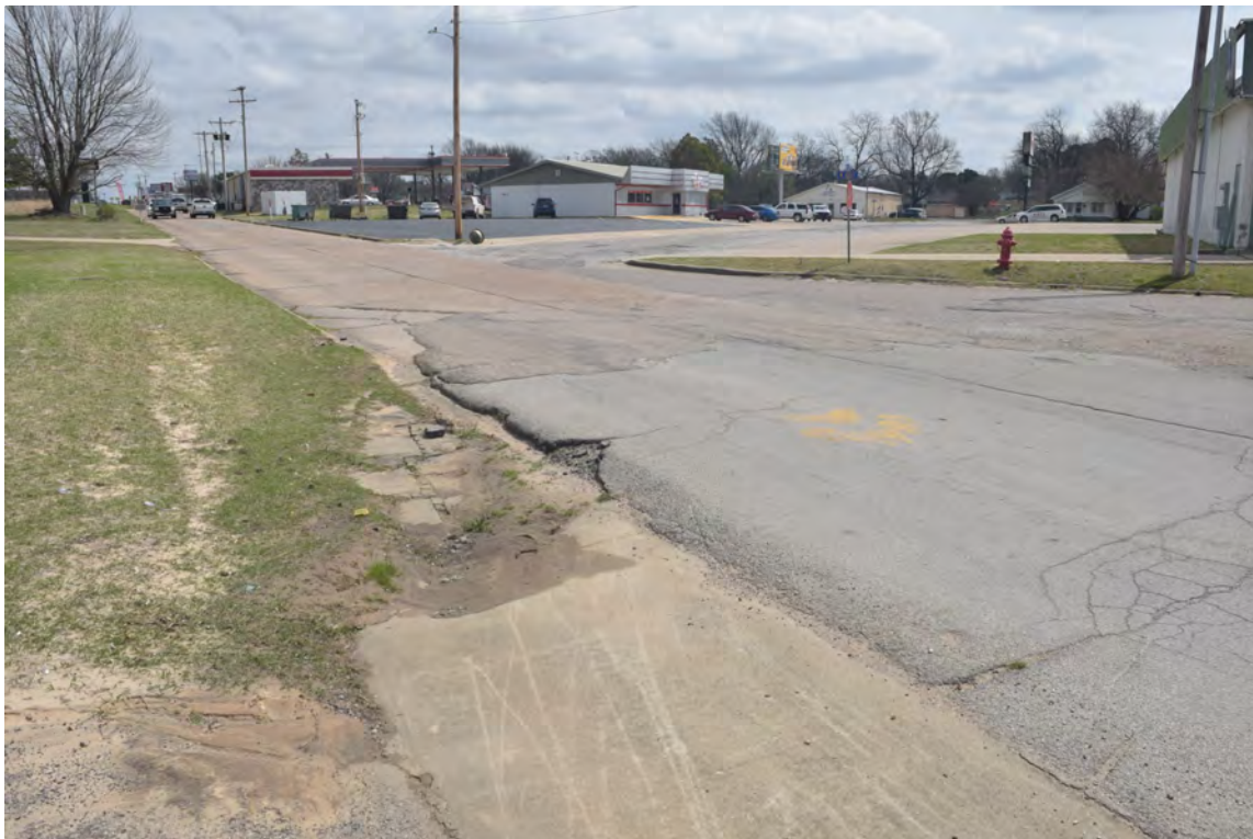
Photo 6: East terminus, concrete insertion over sandstone elements; view facing southeast
