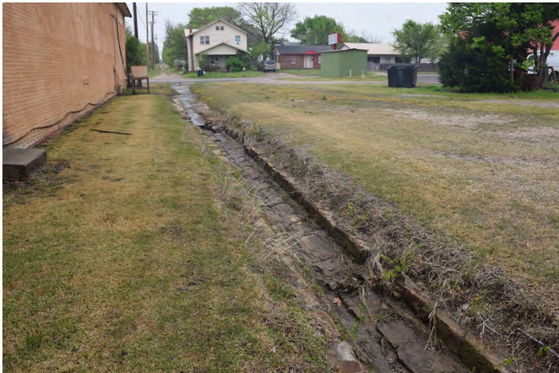
Photo 12: Near east terminus, flat stone bed overlaid with concrete in background; view facing east
