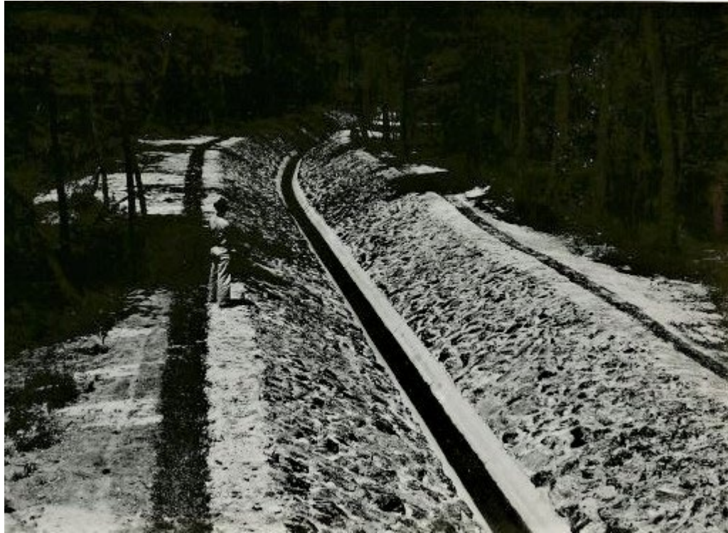
Image 10. Another version of the malaria-control type canal design. This is a 1939 WPA-built example in Alabama. Reproduced from livingnewdeal.com
