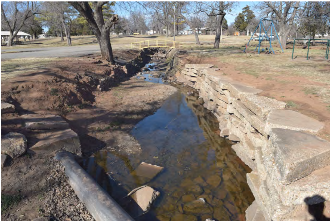
Photo 6: Another curve in canal, concrete wedge replacement material, loss of stonework in evidence, bridge insertion; view facing north
