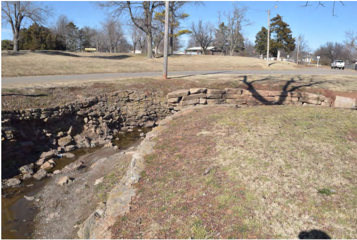
Photo 5: Curve in canal, concrete wedge replacement; view facing north
