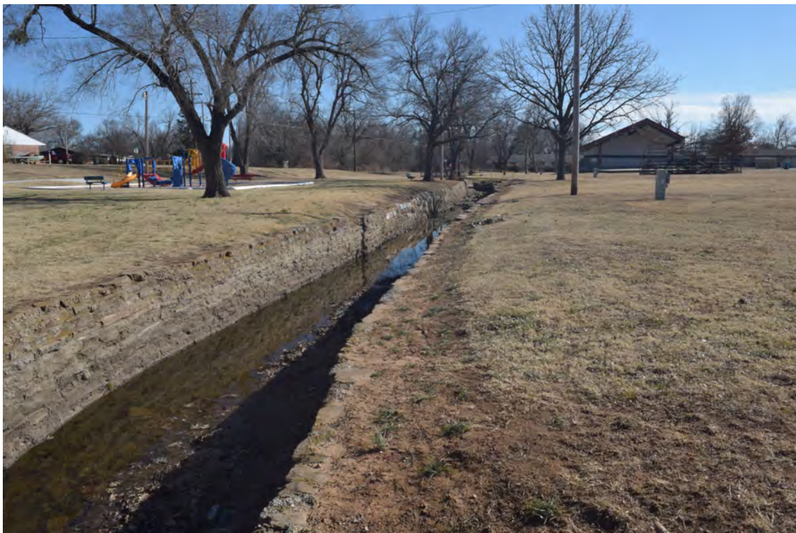
Photo 2: Mortared and coursed stonework, near east terminus; view facing southeast
