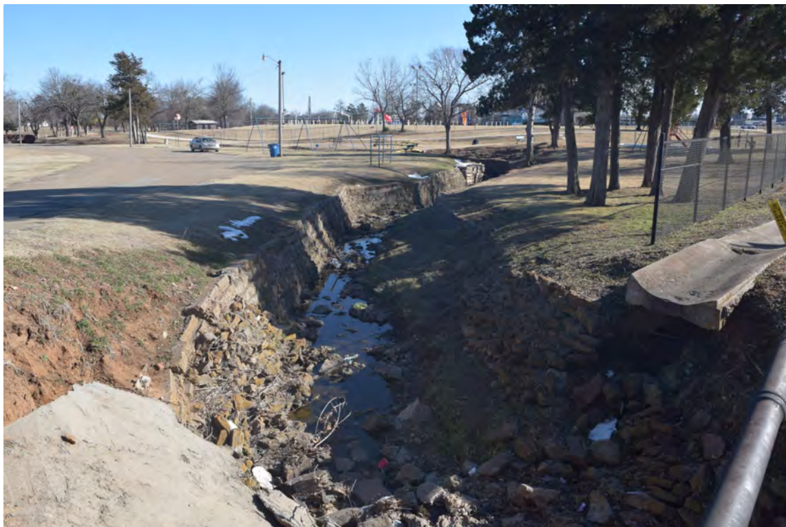
Photo 10: West terminus, mortared and coursed stonework, collapsed stonework, and various insertions near S Little Ave; view facing southeast
