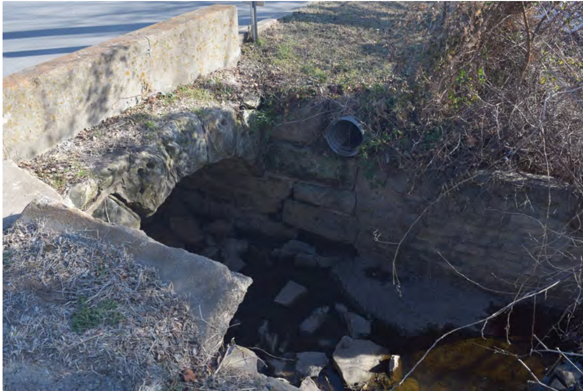
Photo 11: West side of S Little Ave, original stone arch for canal, not present on the east side of S Little Ave; view facing southeast
