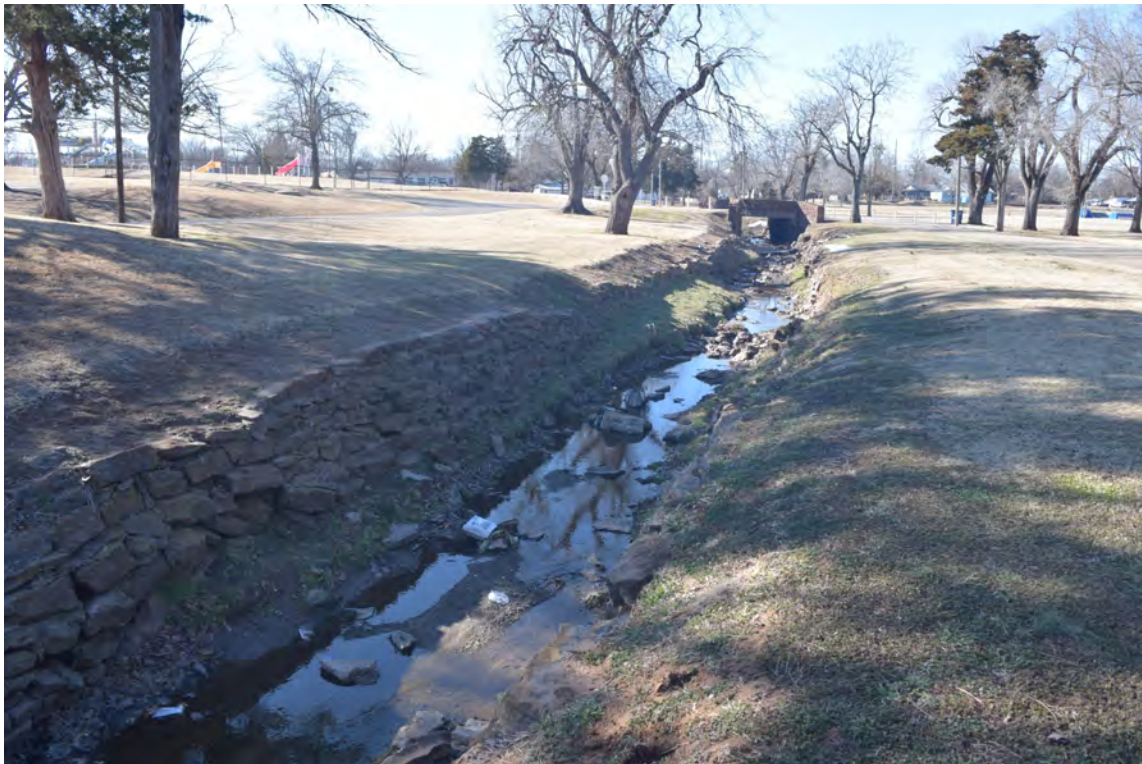
Photo 8: Section displaying coursed, mortared stonework (left bank) and collapsed, removed stonework (right bank); view facing west
