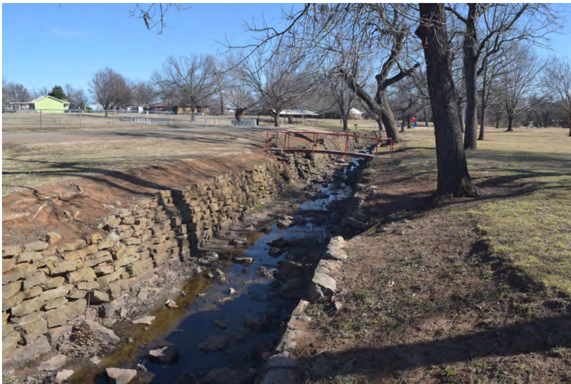
Photo 4: Dry stack stonework and inserted bridge; view facing southeast
