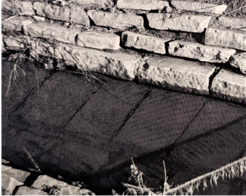
Image 8. Close-up view of a malaria-control type canal design in Checotah, Oklahoma. Note the stepped walls, sloped V-shape bottom and the smaller U-shape down the center of the canal. Reproduced from Leaning on a Legacy by Marjorie Barton.
