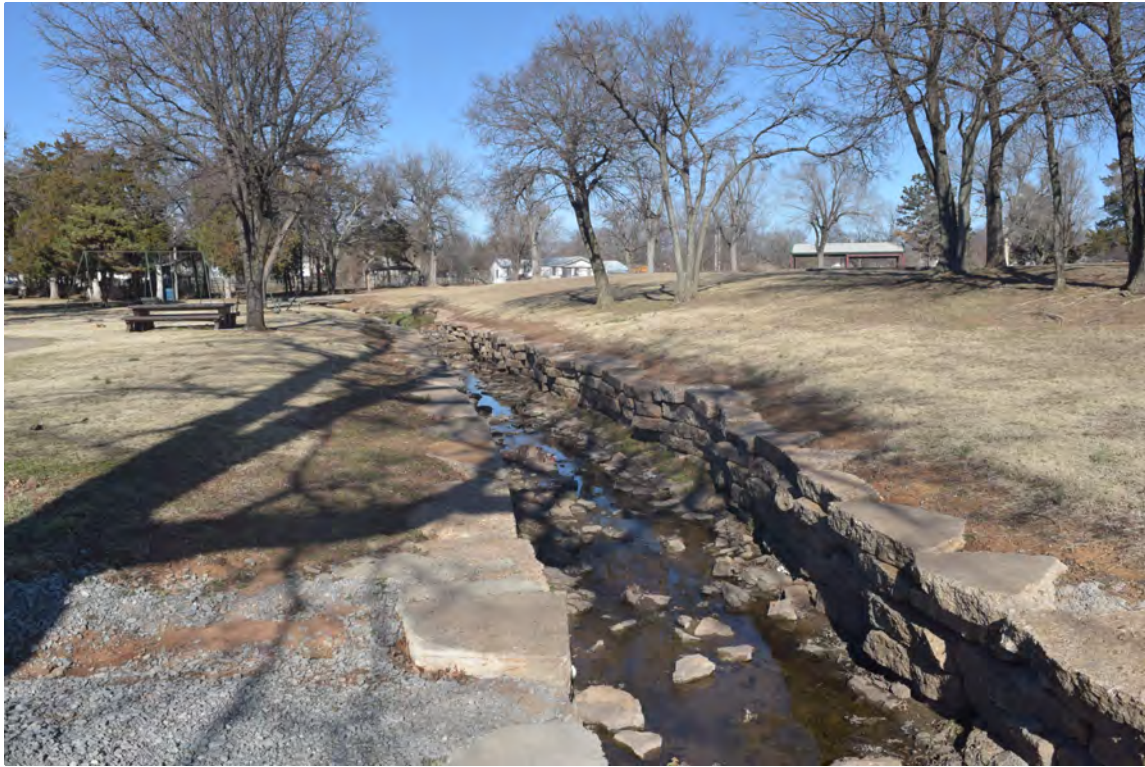
Photo 7: Section of mostly concrete wedge replacement, approximately the middle of Memorial Park; view facing north
