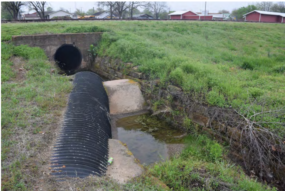
Photo 2: North terminus, detail of water diversion feature; view facing southeast
