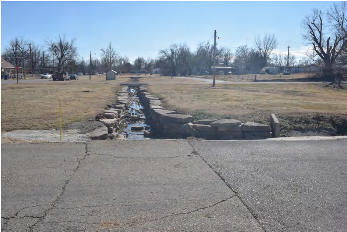
Photo 8: Crossing of waterway at E Oak Street; the section of the canal between E Ash Street and E Oak Street has been fully replaced with piled concrete wedges; view facing south
