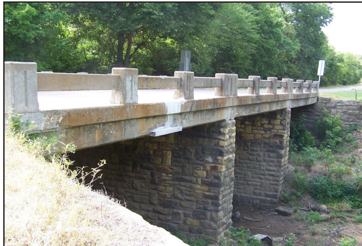
Keel Creek Bridge, Coal County
