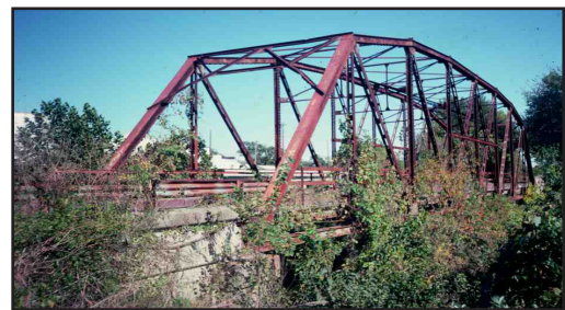
Rock Creek Bridge, Pittsburg County
