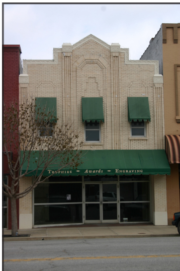
Enid Downtown Historic District, Garfield County
