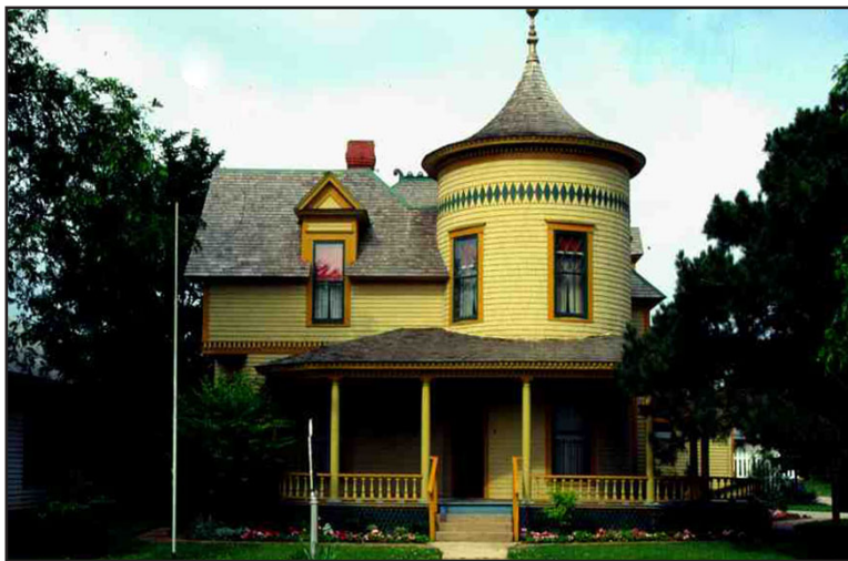
Moore-Lindsay House, Cleveland County
