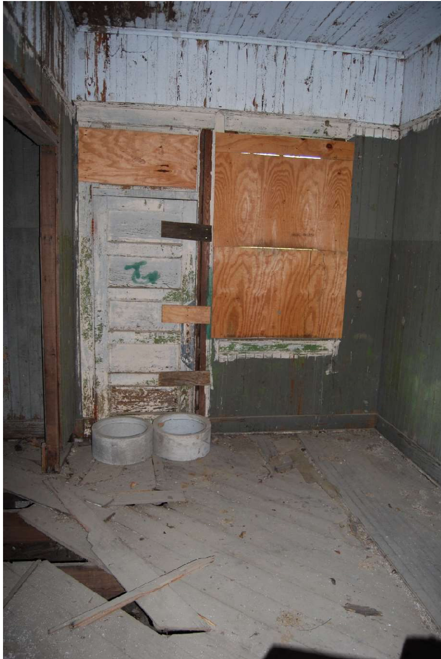
Figure 5: Interior view showing wood door with five horizontal panels. Photograph by Matthew Pearce, OKSHPO.
