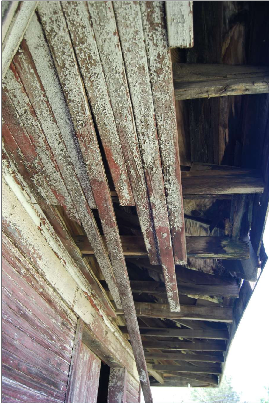
Figure 3: Close up of tongue and groove soffit remnants. Photograph by Matthew Pearce, OKSHPO.
