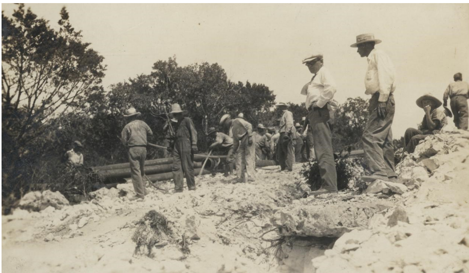
Laying an oil pipeline (21639.5, OHS Photograph Collection, OHS).
