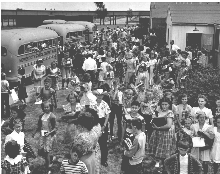
Schoolchildren had to use old Tinker facilities because the size of the school district grew so rapidly (2012.201.B0149.0804, OPUBCO Collection, OHS).
