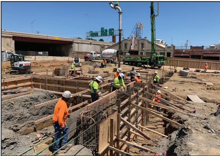
Nabholz Construction builds the footings in preparation to pour the foundation for OKPOP.
