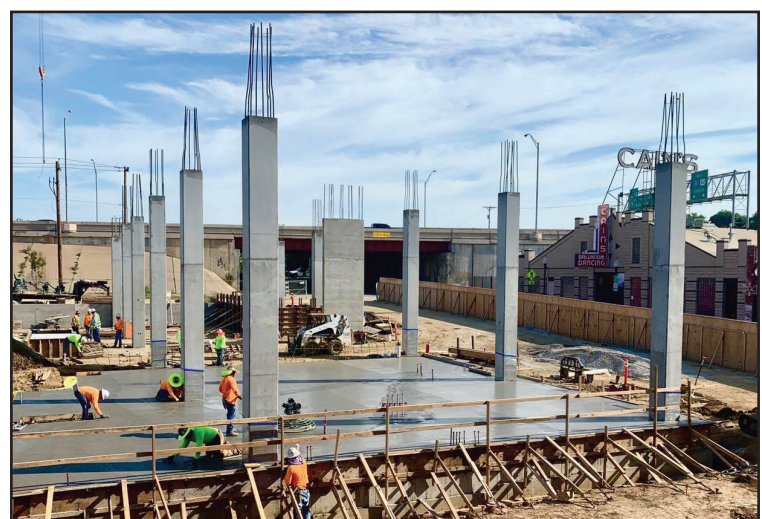
The concrete slab and building pillars forming the first-floor footprint of OKPOP.
