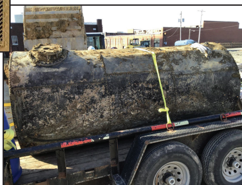
One of two fuel tanks discovered at the OKPOP construction site as excavation began.
