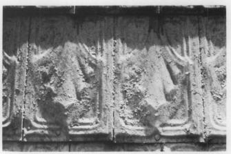
Tin shingles, commonly embossed to imitate wood or tile, or with a decorative design, were popular as an inexpensive, textured roofing material. These shingles  $8^3/_8$  inch by  $12^1/_2$  inch on the exposed surface) were designed with interlocking edges, but they have been repaired by surface nailing, which may cause future leakage. (Ballard House, Yorktown, Virgina, photo by Gordie Whittington, National Park Service)
