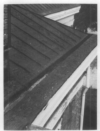
Repeated repair with asphalt, which cracks as it hardens, has created a blistered surface on this sheet-metal roof and built-in gutter, which will retain water. Repairs could be made by carefully heating and scraping the surface clean, repairing the holes in the metal with a flexible mastic compound or a metal patch, and coating the surface with a fibre paint. (Roane County Courthouse, Kingston, Tennessee, photo courtesy of Building Conservation Technology, Inc.)
