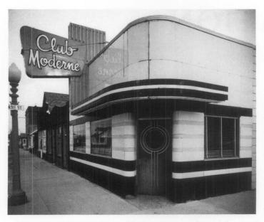
Fig. 1. The Club Moderne, Anaconda, Montana, reflects the exceptional historic detailing associated with pigmented structural glass—polished-mirror finish, rounded corners, and horizontal polychrome bands. Photo: Jet Lowe, Historic American Engineering Record.
