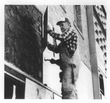
Fig. 16. A worker carefully removes a large glass panel by placing a small piece of wood between a flat prying bar and the glass, then exerting steady pressure. The majority of panels were removed without damage using this procedure. Photo: Thomas Keohan.
