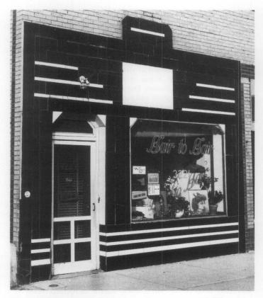
Fig. 15. Owners of this small barber shop, Denver, Colorado, have successfully preserved the historic character of their pigmented structural glass storefront by patching the cracked panels with a dark caulking compound. Photo: Gregory D. Kendrick.
