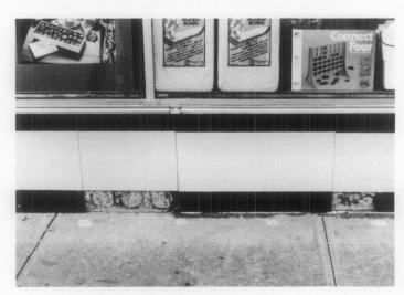
Fig. 14. The vast majority of damaged pigmented structural glass panels are found at ground level, the result of vandalism or improper caulking between the glass panel and the concrete sidewalk. Photo: Thomas Keohan.
