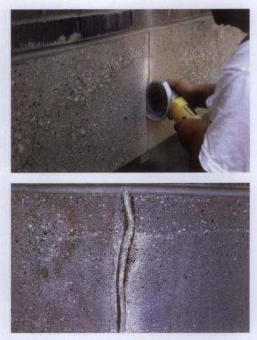
Figure 19. A high-speed grinder ia used to widen a crack in preparation for installation of a sealant. This process is called "routing." After the crack is prepared, the sealant is installed to prevent moisture infiltration through the crack. Although sealant repairs can provide a durable, watertight repair for moving cracks, they tend to be very visible.
