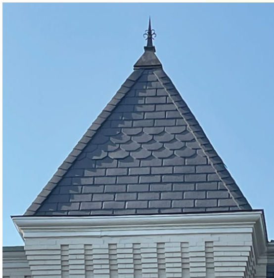
Figure 10a and 10b. Polymer slates offer a choice of shapes but not sizes, limiting their ability to achieve a good visual match for some historic slate. With the size of the polymer slates (Figure 11b) being nearly twice that of the historic slates (11a), the scale of the entire feature is incompatibly altered. The molded edges of this material, which contribute to its ability to replicate slate, would be lost if each shingle was resized by cutting. Photo: John Sandor, NPS.
