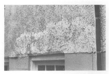
Fig. 14. This poorly executed patch is not the work of a professional plasterer. While it may serve to keep out water, it does not match the original surface, and is not an appropriate repair for historic stucco. Photo: Betsy Chittenden.
