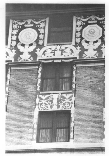
Fig. 11. The Hotel Washington, Washington, D.C. (1916–1917), is notable for its decorative **sgraffito** surfaces. Stucco panels under the cornice and around the windows feature classical designs created by artists who incised the patterns in the outer layer of red-colored stucco while still soft, thereby exposing a stucco undercoat of a contrasting color. Photo: Kaye Ellen Simonson.
