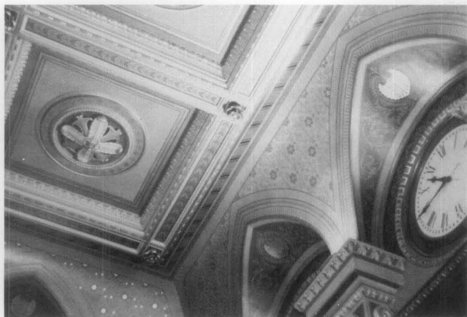
Figure 15. The decorative work on the walls and ceilings of the Senate Chamber, Providence, Rhode Island, City Hall (1875) is a rich combination of paint and gilding on ornate plaster features. It was carefully restored in 1975. Photo: Kate Gilliat. © Providence Preservation Society.
