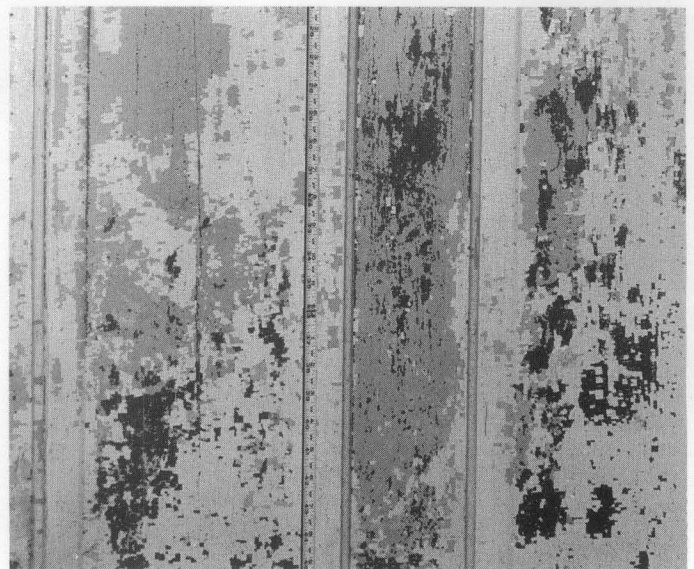
Figure 11. A dark layer can be seen beneath the flaking lighter paint on these raised field panels. Depending on the project work goal and the period of the building's history being interpreted, any one of the paint layers could be duplicated in repainting. National Park Service files.
