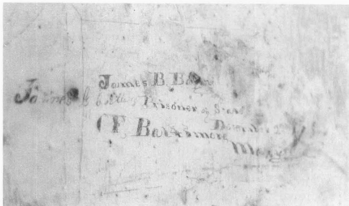
Figure 12. When discovered, important examples of history such as this pencilled Civil War graffiti should be preserved. A conservator can easily clean the area, then apply a protective coating. The history this hand-written message possesses is well worth the sacrifice of surface uniformity, even if it interrupts a freshly painted surface. Photo: Kaye Simonson.
