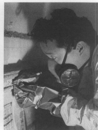
Figure 23. Methylene chloride fumes can be deadly, so protecting the worker is imperative. Left: a hooded, air-fed unit. Right: a vapor mask with organic solvent cartridges. Photo left: William Adair. Photo right: Lonnie J. Hovey, AIA.
