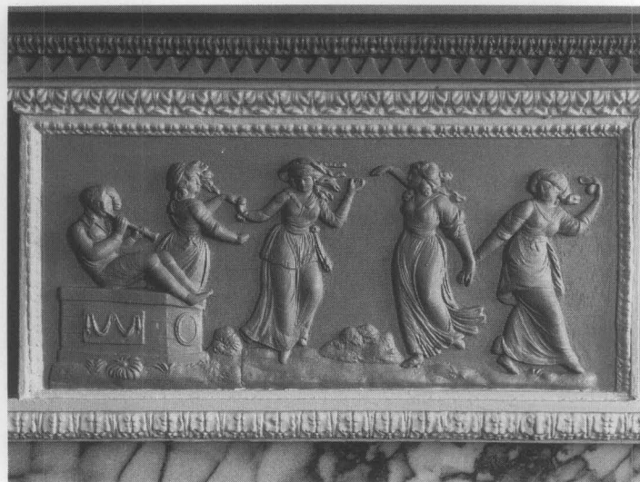
Figure 21. The same theme on two early mantelpieces, A Country Dance , dramatically illustrates the visual difference between cleaned and uncleared composition ornament. When old paint layers are removed, the exquisite detailing is revealed. Left: George Read II House, 1801-1803, New Castle, Delaware; Right: First Harrison Gray Otis House, 1796, Boston, Massachusetts. Photo left: Gold Leaf Studios, Inc. Photo right: David Bohl. Courtesy, Society for the Preservation of New England Antiquities.
