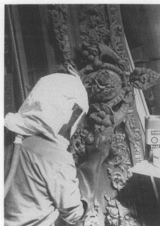
Figure 23. Methylene chloride fumes can be deadly, so protecting the worker is imperative. Left: a hooded, air-fed unit. Right: a vapor mask with organic solvent cartridges. Photo left: William Adair. Photo right: Lonnie J. Hovey, AIA.
