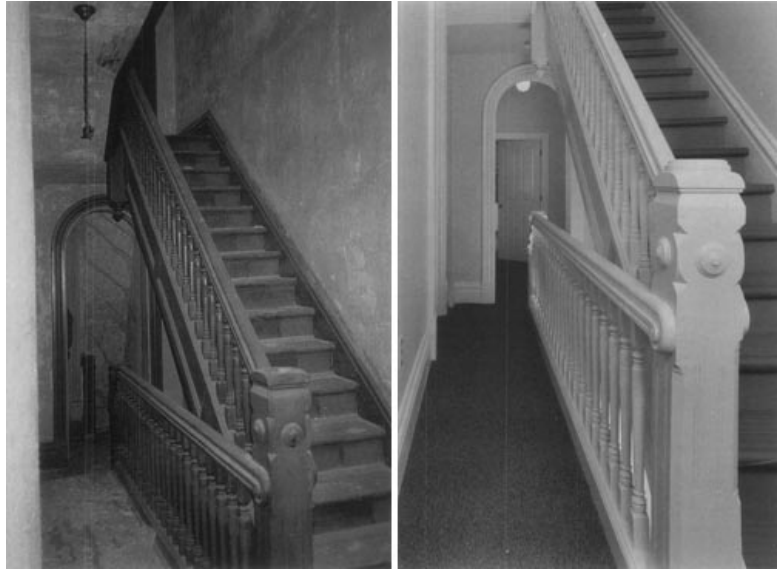
A large-scale historic rehabilitation project incorporated sensitive lead-hazard reduction measures. Interior walls and woodwork were cleaned, repaired, and repainted and compatible new floor coverings added. The total project was economically sound and undertaken in a careful manner that preserved the building's historic character. Before:left, after:right. Photos: Landmarks Design Associates.
