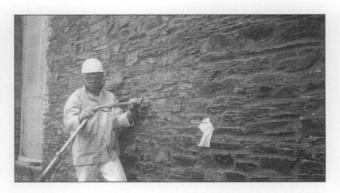
17. The internal grout injection of rubble walls can improve seismic capacity. Care must be taken in formulating the mortar grout and repairing the area where injection occurs. Photo: Architectural Resources Group, San Francisco.
