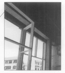
14. The use of a steel moment frame to support the large open storefront during a rehabilitation eliminated the need to place diagonal braces or other intrusive supports in a highly visible area of a historic building. Photo: David Look.
