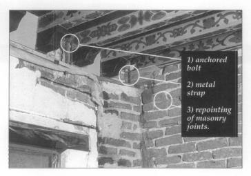
11. Limited intervention should correct obvious structural deficiencies, such as tying vulnerable elements together and repointing masonry. Seen here is 1) anchored bolt, 2) metal joist strap, and 3) repointing and reinforcing masonry joints. Upon replastering and painting these reinforcements will not be visible. Photo: Historic Preservation Partners for Earthquake Response.
