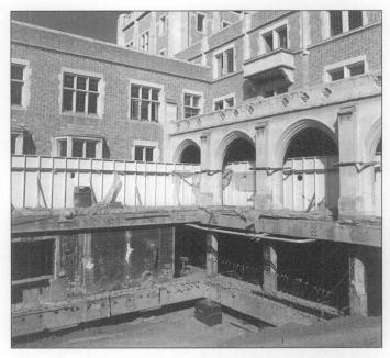
8. Full seismic restructuring to ensure that buildings survive a major earthquake with a minimum of damage may involve extensive reinforcement. Upon completion, the changes to this ca. 1932 Gothic Revival building to add base isolation at the foundation were not visually apparent. Photo: © Jonathan Farrer, courtesy University of California at Los Angeles (UCLA), Capital Programs.
