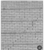
3. Forces from moderate to serious earthquakes caused a) the untied gable to fail, b) the first floor to collapse c) cracks from the pounding effect of adjacent buildings, and d) and diagonal cracks in exterior masonry between windows to form. Photos: David Look.
