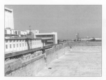
15. The use of fiber composite materials can enhance the shear capacity of existing structural components -beams, columns, and surface elements, such as walls and floors. In this roofing application, the existing roof diaphragm is being strengthened and there is additional benefit to the shear reinforcement of the parapet wall. Photo: The Crosby Group.
