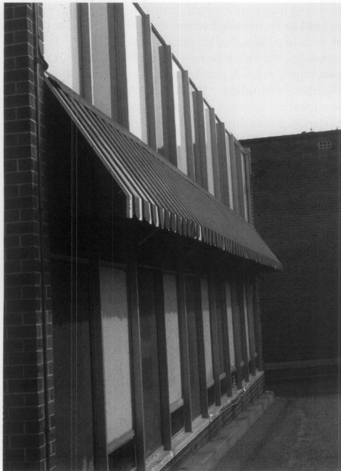
Figure 15. This 1950s-era dry cleaner has an aluminum awning that, with its vertical pattern and alternating stripes, complements the facade's porcelain enamel panes and aluminum mullions. The awning forms an essential element of the building's historic character.
