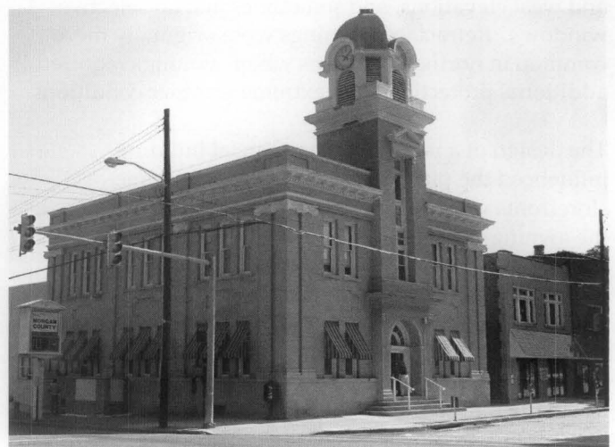
Figure 18. (Above) When the county clerk in Morgan County, West Virginia, was looking to reduce glare in the courthouse offices she located a 1940s photo showing sets of awnings on the first floor. (Below) Using the historic photos as a guide, new awnings with a similar shape and stripe pattern were installed increasing the comfort of employees and protecting county records from direct sunlight. Above photo: Frances Widmeyer and Debra Kesecker.
