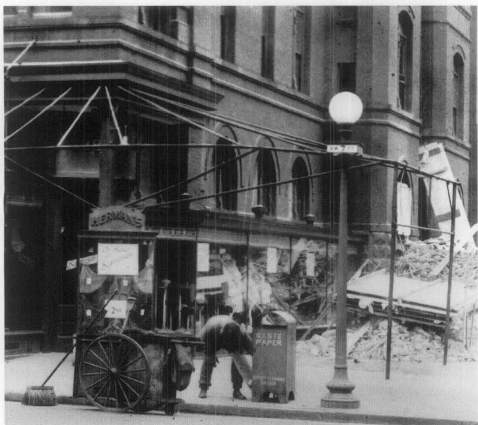
Figure 5. During the second half of the 19th century, iron plumbing pipe became a popular material for fixed awning frames. Here, a pipe frame without its canvas cover extends around the corner of a building in Washington, D.C. Photo: Library of Congress, Prints and Photographic Division, LC-USZ62-121160.
