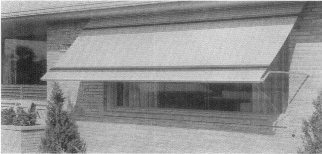
Figure 14. The years after World War II saw the widespread adoption of aluminum awnings on both storefronts and residences. Operable aluminum awnings incorporated a spring-loaded roller into the frontbar.
