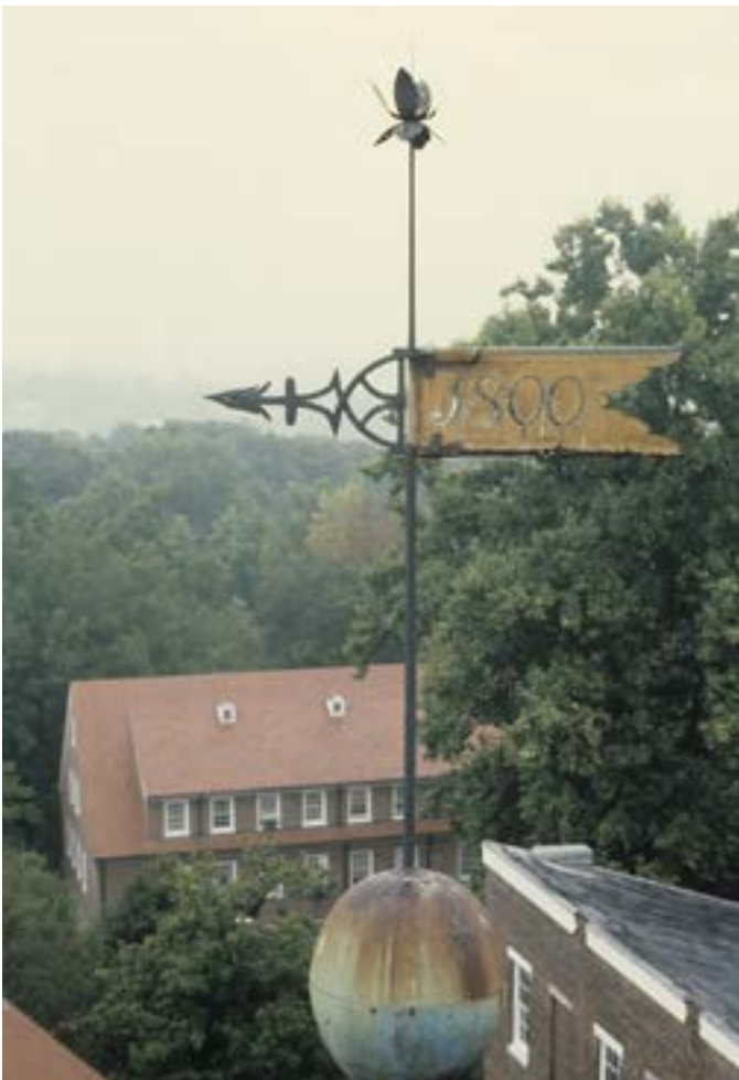
Figure 8. Church steeples, roof turrets, and chimneys were identified early on as being susceptible to lightning strikes. Finials, weathervanes, and other such ornamentation in these locations could often serve as lightning rods when connected to down conductors and grounds. The cupola on the Home Moravian Church in Winston-Salem, North Carolina, is an excellent example. Old Salem, Inc., has a number of Moravian buildings where early lightning protection systems are still in place. Photo: Sunni L. Goodson.
