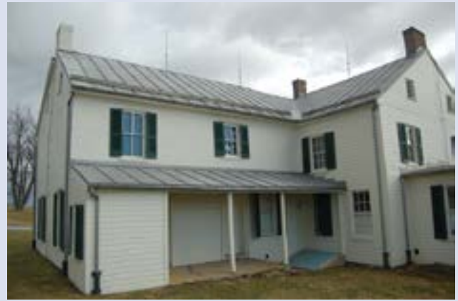
Figure A. Rear view of the Mumma House showing three of the four tall reproduction lightning rods placed close to the same locations as the historic ones, which were too deteriorated to reuse. Running down the left side of the house below the chimney is one of the two historic down conductors, which were saved in place and bonded to the new system. Photo by author.
