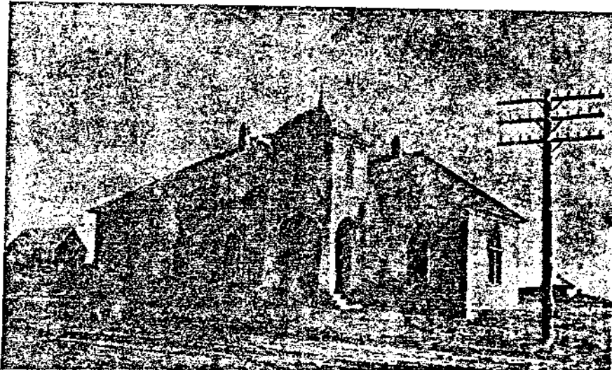
Methodist Church (Destroyed)
