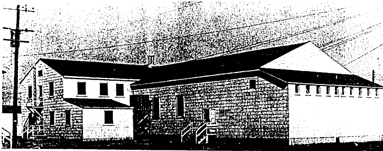
Temporary buildings transported from Amarillo Air Field at the end of World War II and used as a student recreation hall until 1965.
