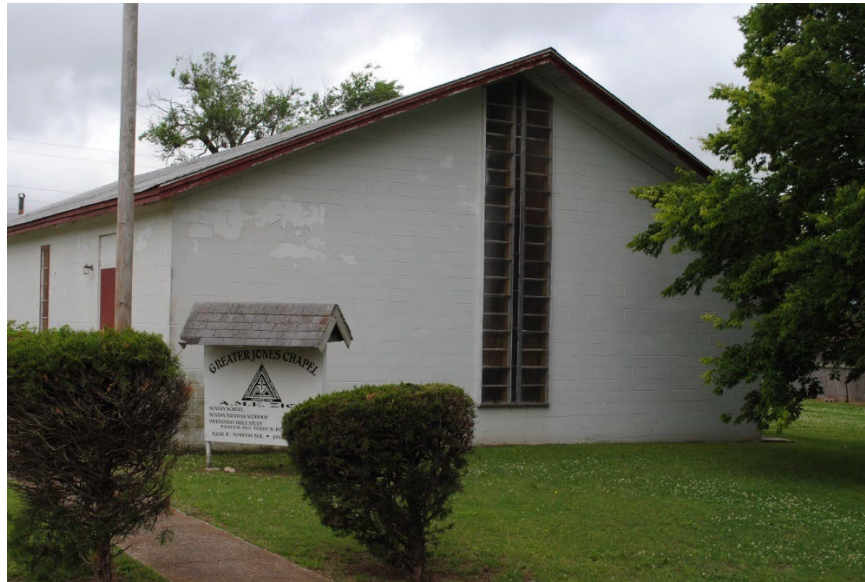
Figure 9: Greater Jones Chapel at 1226 East Smith Street displays some modest Modern Movement-style influences, most notably tall vertical window openings at the gable ends.
