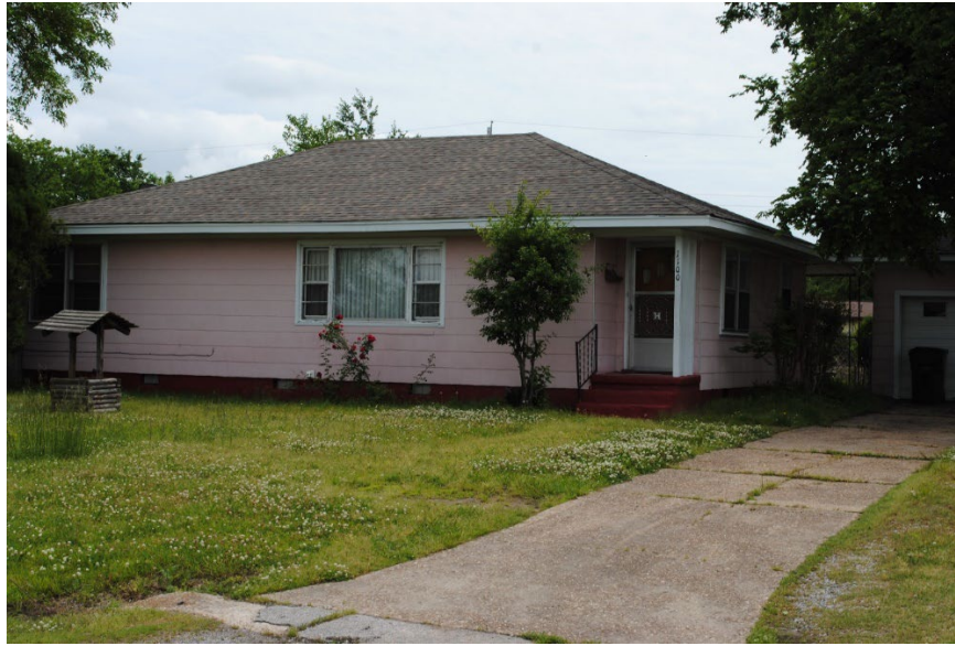
Figure 4: This one-story single-family dwelling at 1100 East 1 st Street retains a high degree of integrity and displays several features indicative of the Minimal Traditional style, including a modest, square-shaped footprint, intermediate-pitched hipped roof, and modest exterior detailing. The property is also notable for having a detached, one-car garage (right).
