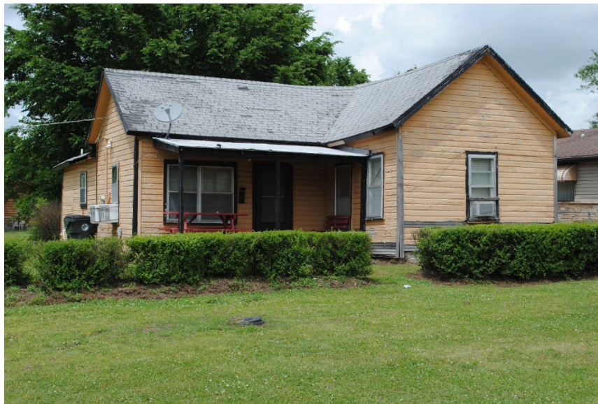
Figure 2: This house at 1101 East 1 st Street is an excellent local example of a cross-gabled, Folk-style residence. Note the shed-roofed porch within the “L” of the two gabled wings. Two entrances are under the porch roof. Notable exterior materials include painted wood siding and a stone foundation.
