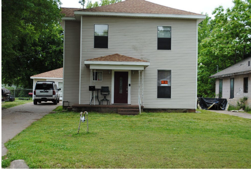
Figure 5: The William Shealey House at 1022 East 2 nd Street was previously identified as an important local example of the American Foursquare house type. Note the non-historic siding, windows, and altered front porch.
