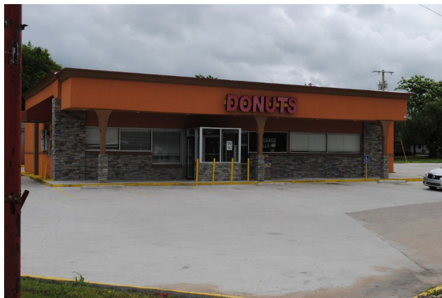
Figure 7: This c. 1975 commercial building at 811 North Wood Drive was modified in c. 2021, when it became a donut shop. Notable modifications include new stone veneer and alterations to the roofline and storefront windows.
