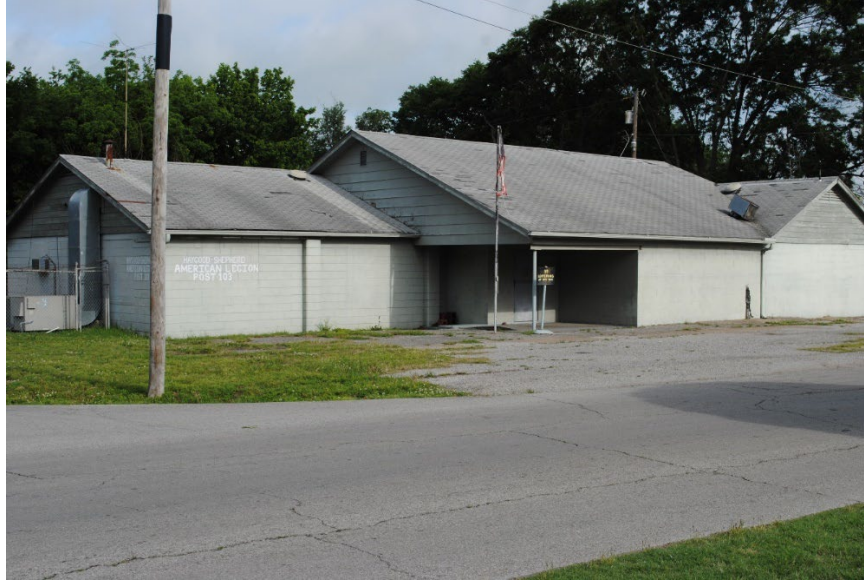
Figure 8: The Haygood-Shepherd American Legion Post (800 North Wilson Street) has a concrete block exterior and cross-gabled roof. The east (front) elevation was modified to its current configuration by 1980.
