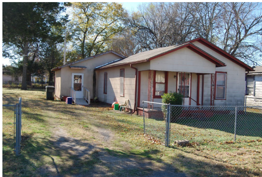
Figure 3: Several common exterior modifications were observed throughout the survey area, including replacement exterior materials, windows, and doors. This c. 1960 Craftsman/Bungalow-style single-family dwelling at 1118 East 3 rd Street retains most of its historic exterior materials but has a significant rear addition that was constructed sometime between 1995 and 2003.
