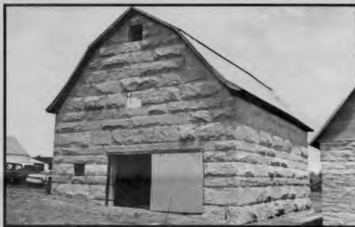
West Barn, J. P. Tipton Farmstead, Kay County
