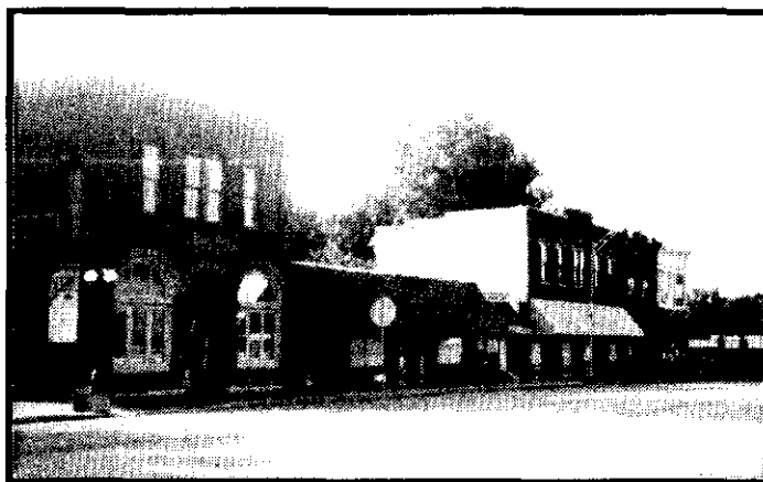
Historic Buildings in downtown Perkins
