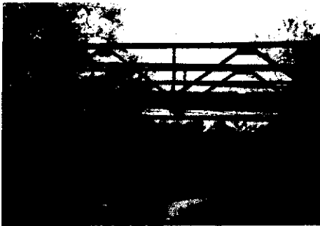
Little Deep Fork Creek Bridge, Bristow
