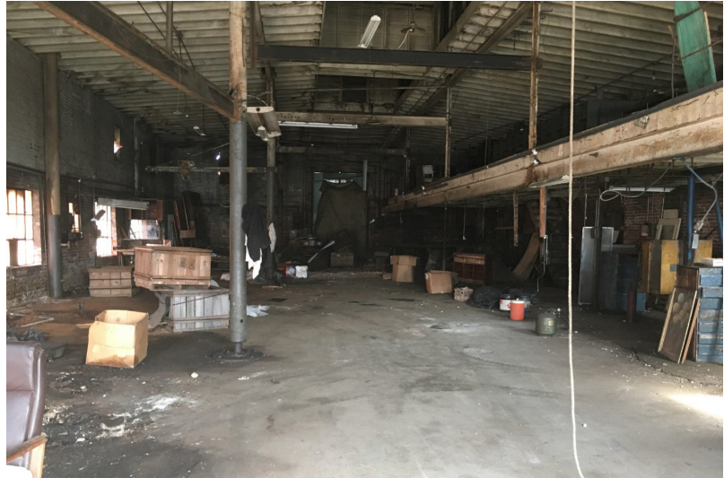
Although currently covered by a non-historic metal roof, interior investigations of the Anderson Building in the Sapulpa Downtown Historic District revealed the historic roof structure with monitors remained intact. Photo: OK/SHPO.
