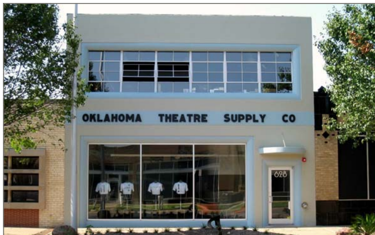
Oklahoma Theatre Supply Co Building, Oklahoma City, Oklahoma County
