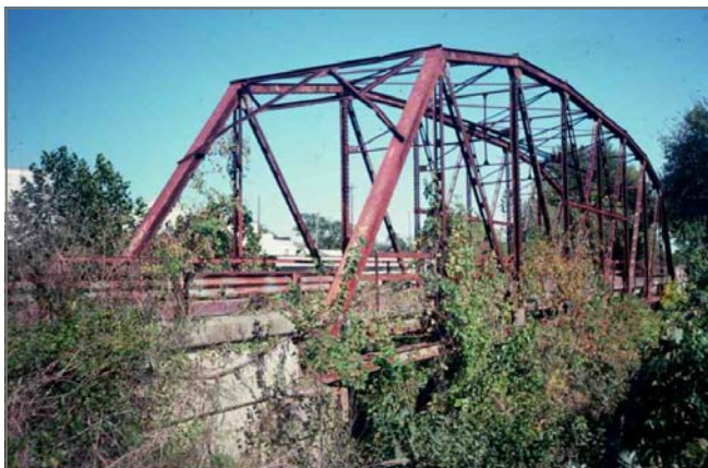
Bridge #18 at Rock Creek, Sapulpa, Creek County
