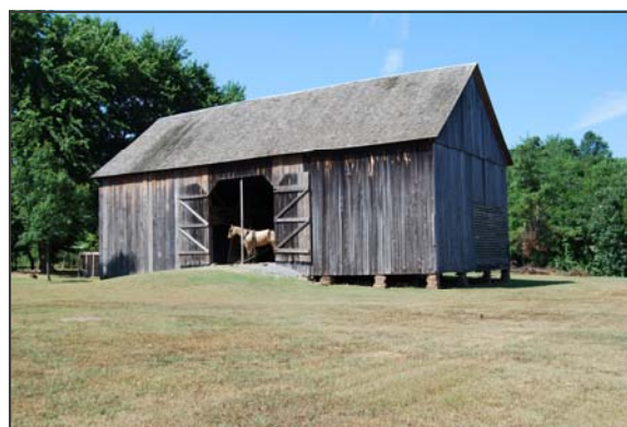
Peter Conser House, Barn, Heavener, LeFlore County
