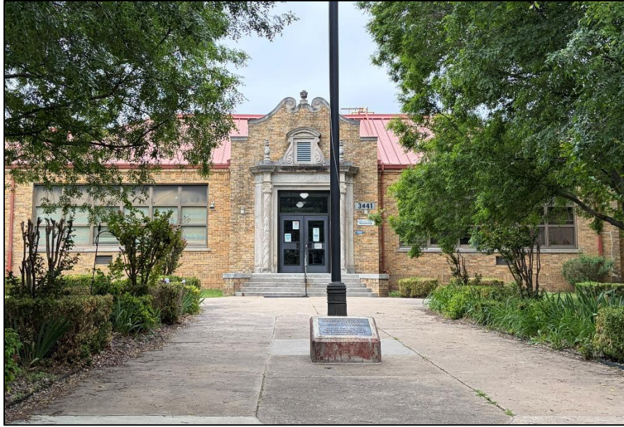
Figure 5. The Spanish Revival style entrance to the Sequoyah School. Photograph by Loggia Preservation, 2026.
