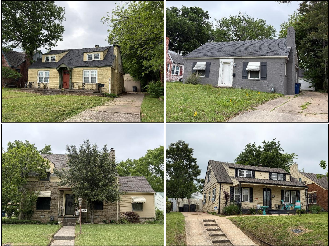
Figure 4. Examples of the Colonial Revival style in the survey area. Clockwise from upper left: 3316 East Archer Street; 3314 East Admiral Court; 3506 East Archer Street; 3503 East Easton Street. Photographs by Loggia Preservation, 2026.
