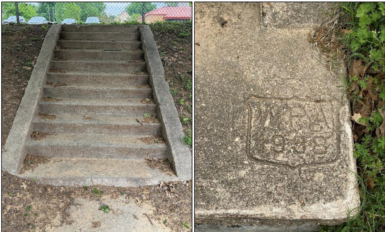
Figure 24. Concrete staircase completed by the WPA in 1938. Concrete staircase completed by the WPA in 1938. WPA-marked features include two staircases and a short run of concrete steps, all of which lead from the sidewalk on the east side of North Indianapolis Avenue to the Sequoyah School and its field. WPA markings were not observed elsewhere on the property. Photograph by Loggia Preservation, 2026.
