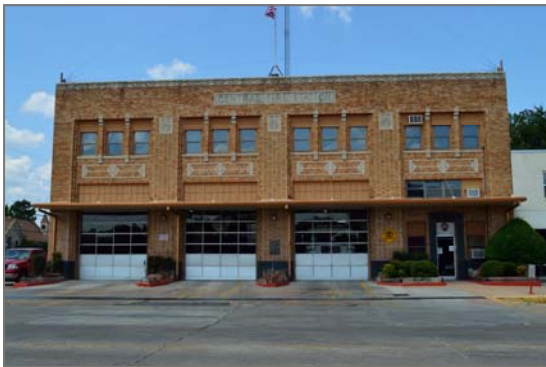
Central Fire Station, Lawton, Comanche County
